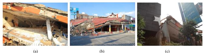
Figure 3. Lack of sufficient bracing and use of strong beams - weak columns
