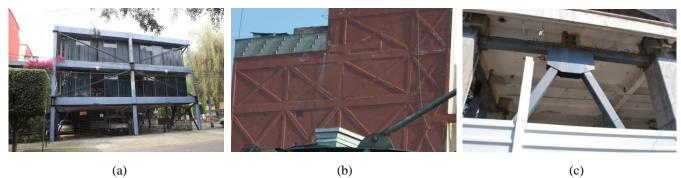
Figure 10. Seismic retrofit of frame buildings with steel braces
