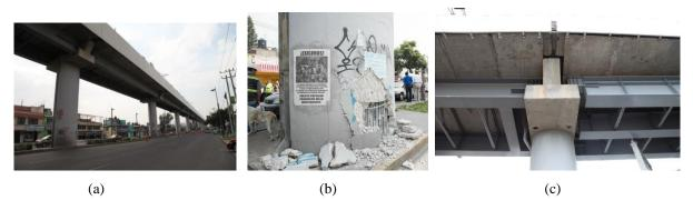
Figure 13. (a) Mexico Metro Line viaduct, (b) plastic hinge forming at the base of a bridge column, (c) longitudinal displacement at deck level and lateral displacement
