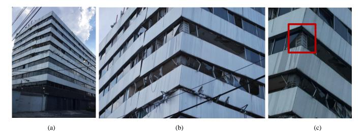
Figure 8. Eight-storey government office building with retrofitted columns following the technique illustrated in Fig. 7 suffered collapse of the 4<sup>th</sup> storey columns
