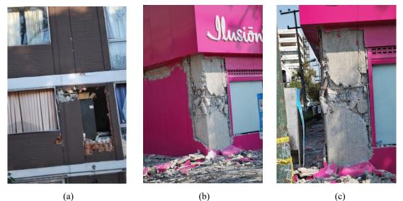
Figure 5. Lack of concrete confinement and buckling restraining ties in pre-1985 buildings
