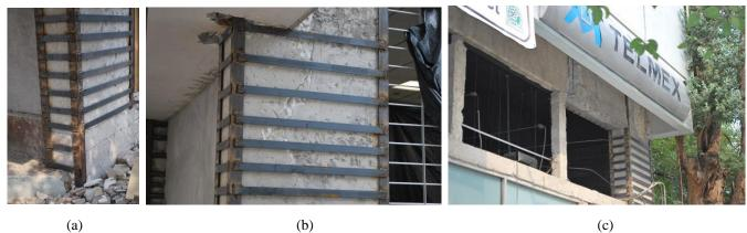
Figure 7. Column retrofit technique commonly used n Mexico City
