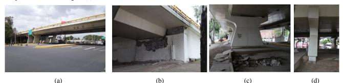
Figure 14. (a) Parallel 5-span underpass, (b) damaged URM abutments, (c) rocking of wall pier, (d) tilting of wall pier
