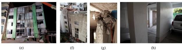
Figure 12. Reinforced concrete buildings with soft stories
