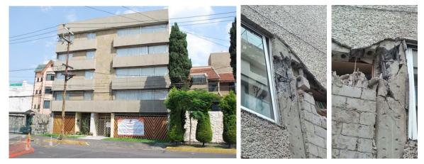
Figure 6. Lack of column transverse reinforcement and short column effect in a post-1985 reinforced concrete frame building with concrete block masonry infill walls
