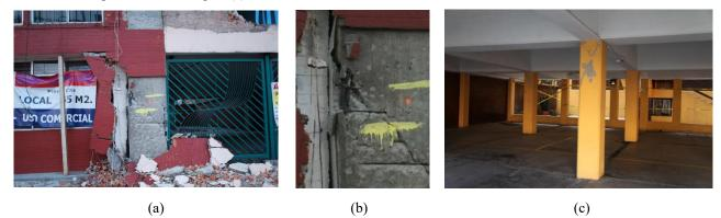
Figure 4. Diagonal tension cracking of first-storey columns due to insufficient transverse shear reinforcement
